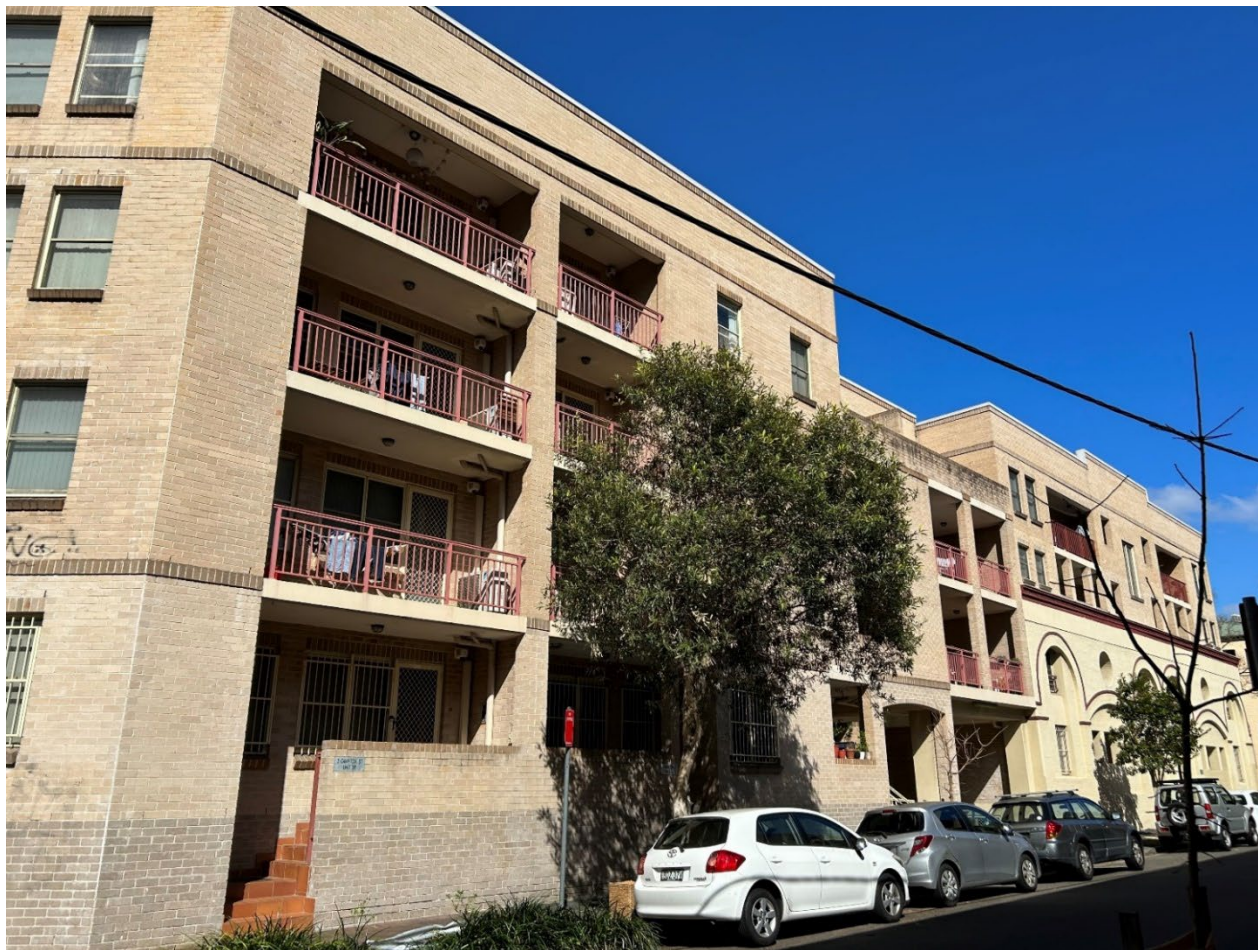
apartment building (23-35 Buckland Street) to south across Grafton Street
