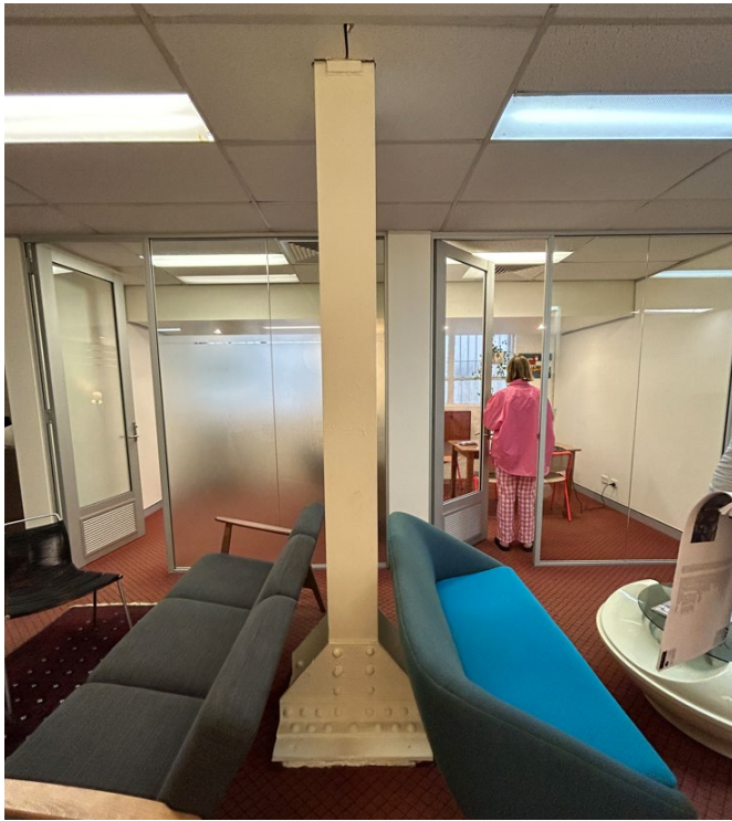
structural columns to be retained
