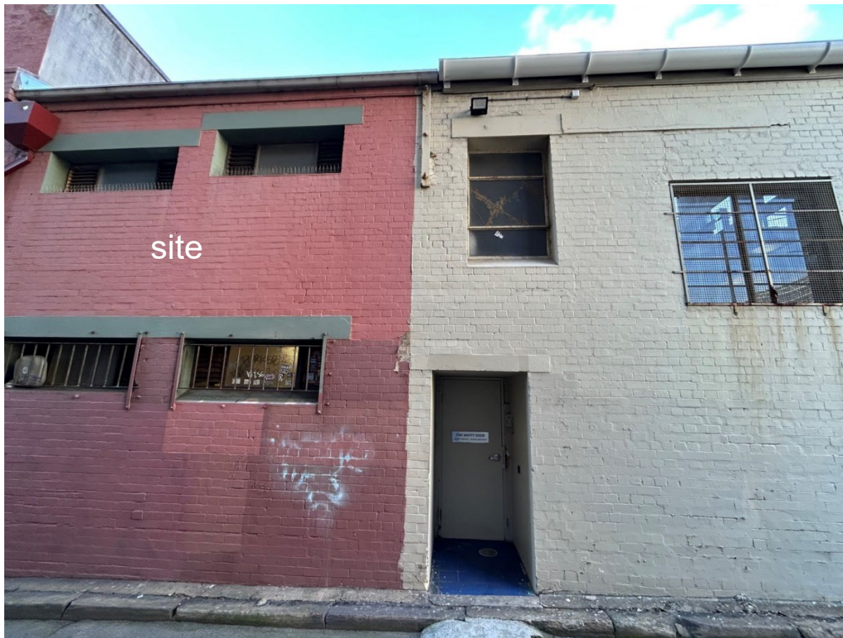
site's emergency egress door to Grafton Lane located on adjoining premises
